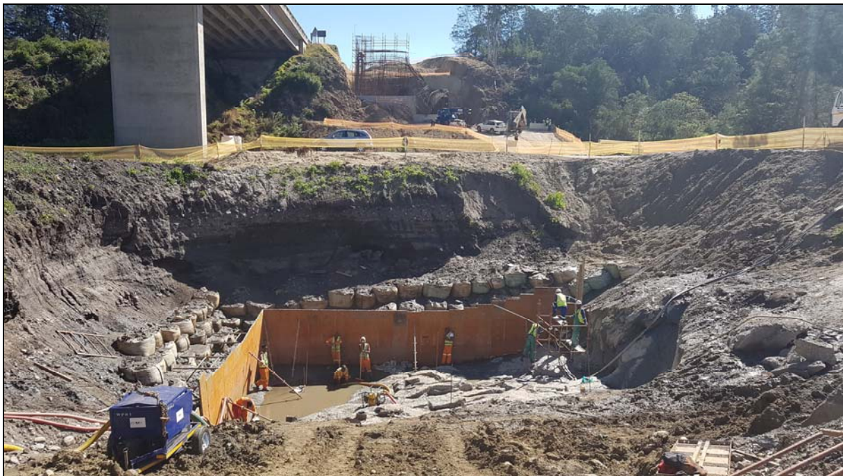
Figure 12: Deep excavations, lateral support and dewatering for bridge pad foundations
